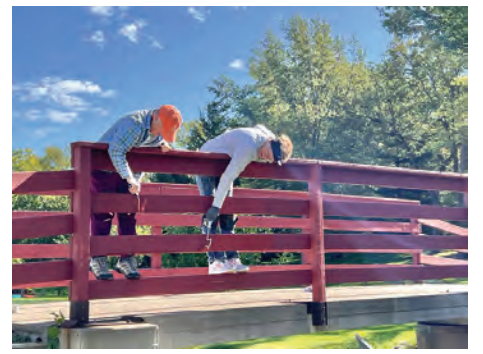
Painting Birch Park Bridge
