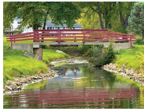
Birch Park Bridge
