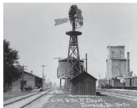
This railyard scene from early Durand history shows the water tank and windmill to replenish the supply for the steam engine and the grain elevator which was a feature of so many small towns in the midwest.
